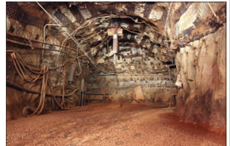
The workshop area on the 4850 Level is now free of water. (Photos courtesy Bill Harlan, Sanford Underground Laboratory.)
